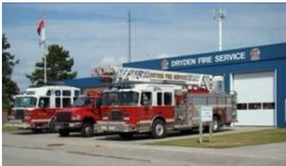
Figure 18. Hall #1 (source: Dryden Fire Service).
